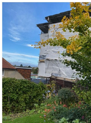
Fig. 1: view from 112 Denton Drive during the work
